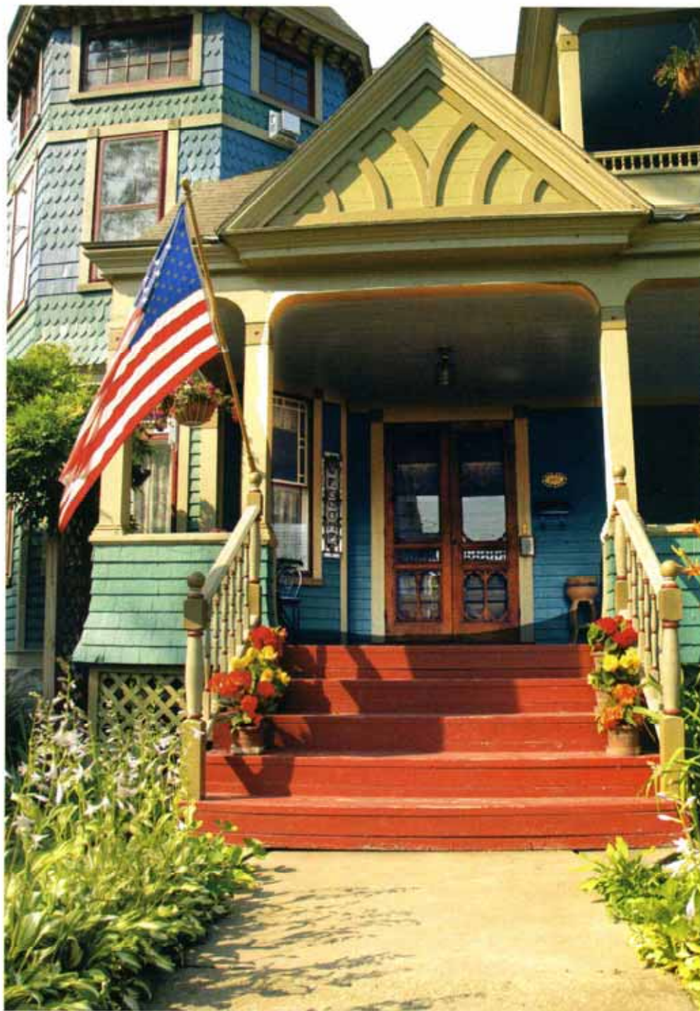
The Trimmer House (circa 1891), a bed and breakfast on East Main Street, Penn Yan
